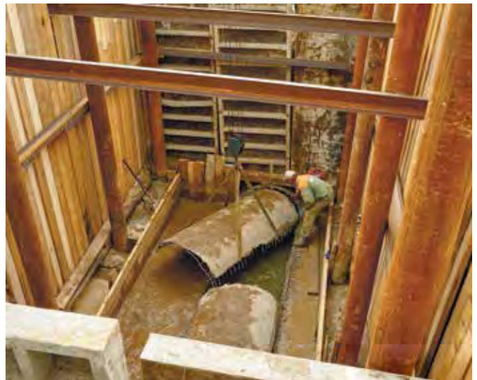
Pic. 2. Opening of the crown of pipelines
