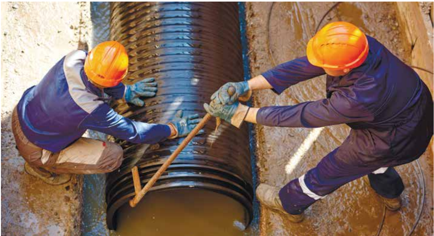
Pic. 4. Screwing-in of thread modules
