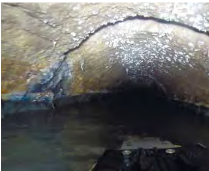
Pic. 1. CCTV of gravity pipeline
