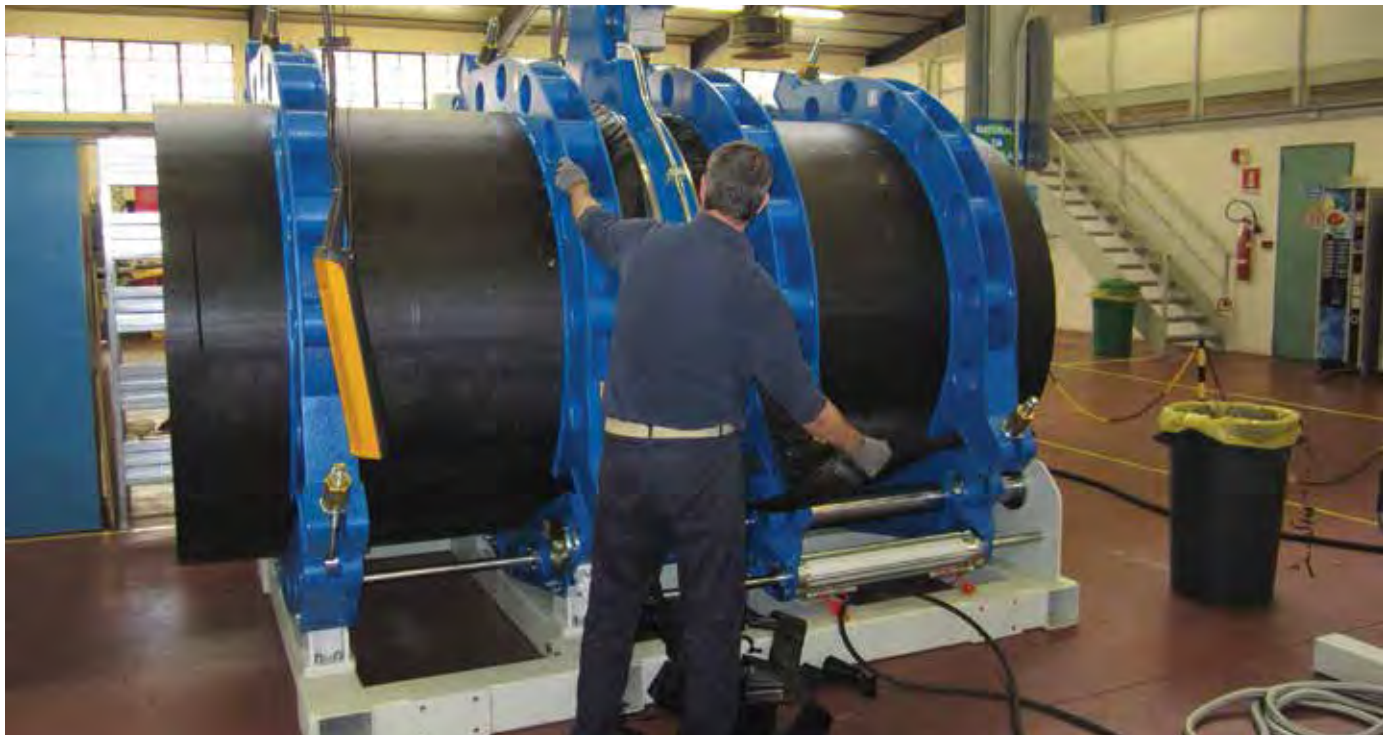
FIG. 6. Welding of 95 mm wall thickness pipe
