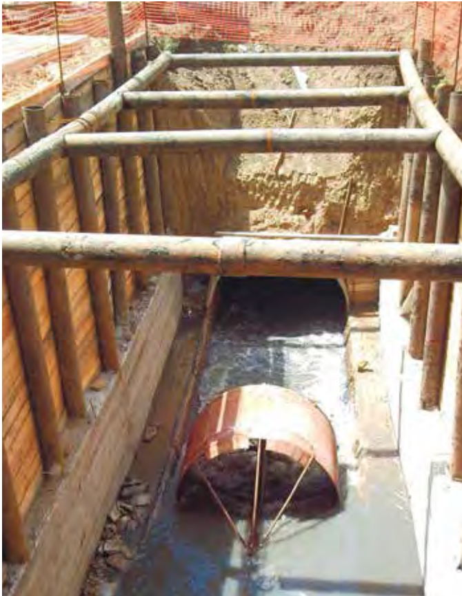
Pic. 3. Pipelines bottom cleaning
