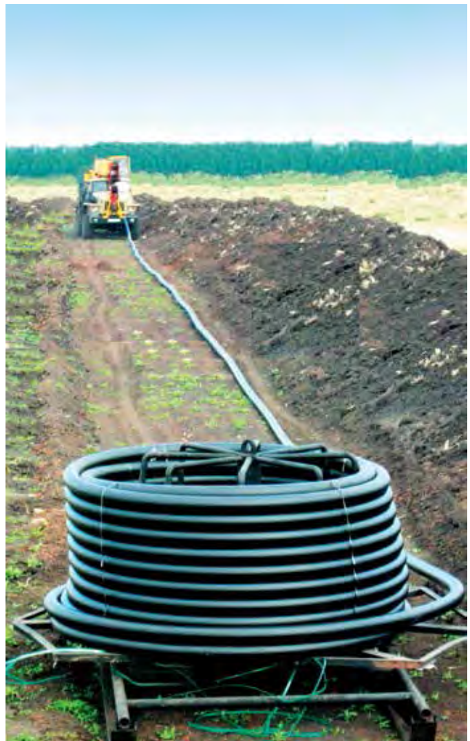
Pic. 2. Uncoiling of Anaconda™ pipe during construction of oil flowline
