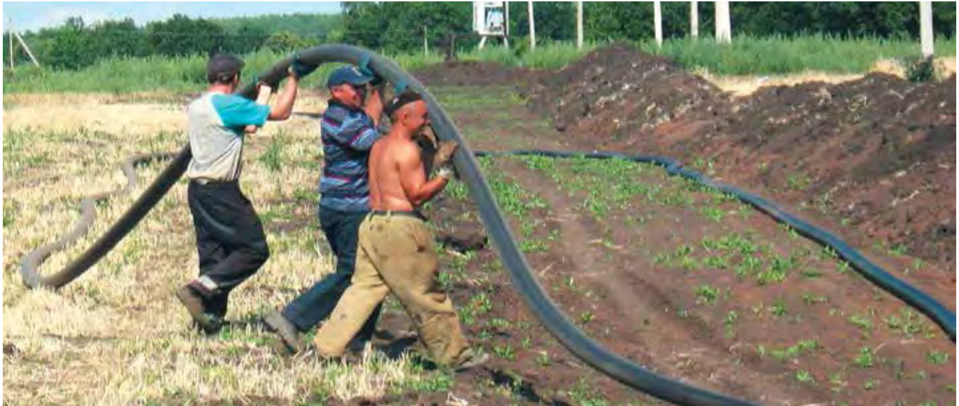
Pic. 3. Oil flowline positioning
