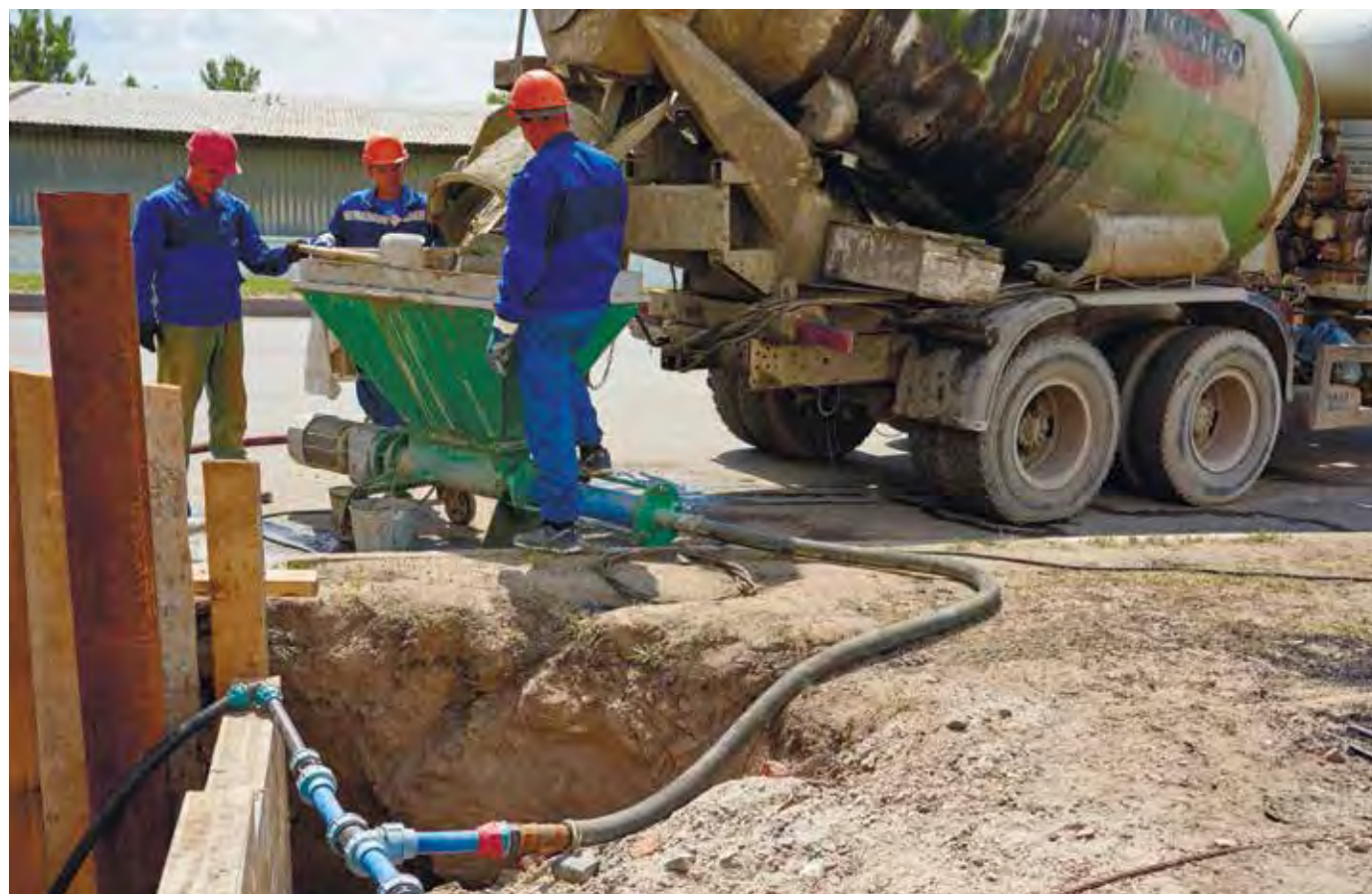
Pic. 5. Filling of the void between the pipes.
