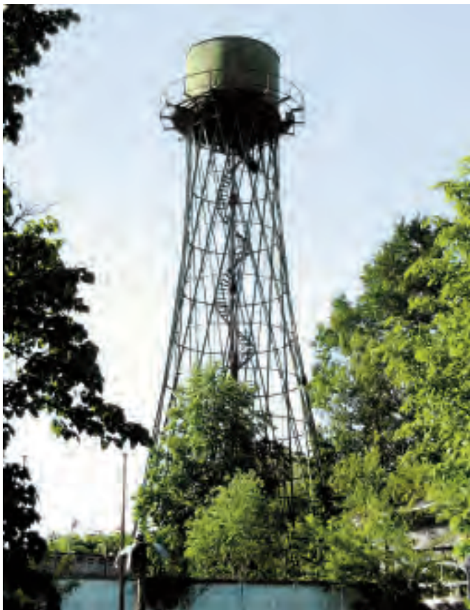
The water tower in Lugovaya village (Moscow Region)
