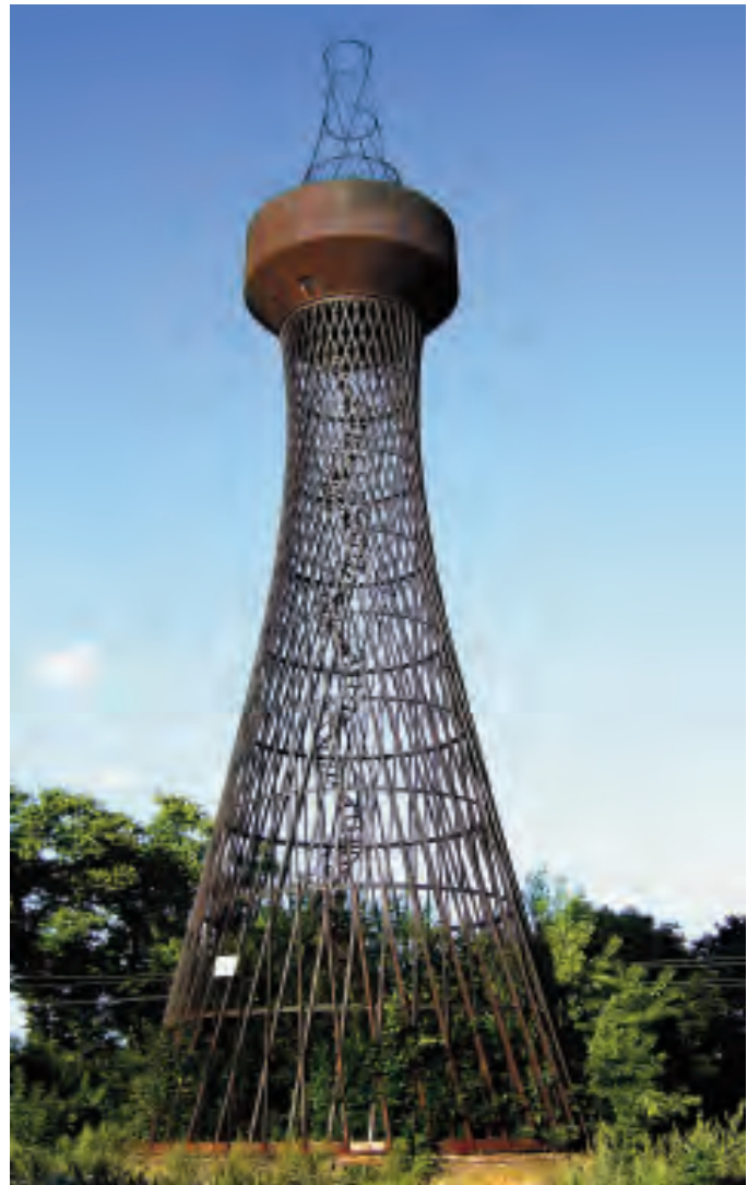
The same Water tower in Polibino village. Lipetsk Region, 2014
