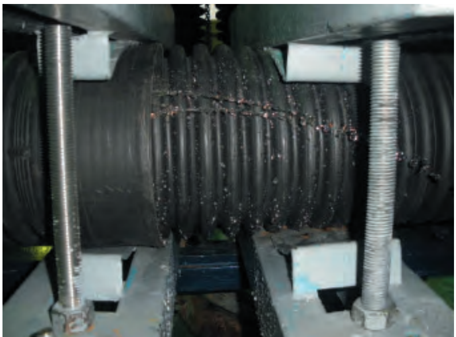
Leaking in-line molded pipe joint during leak testing according to EN 13476-3
