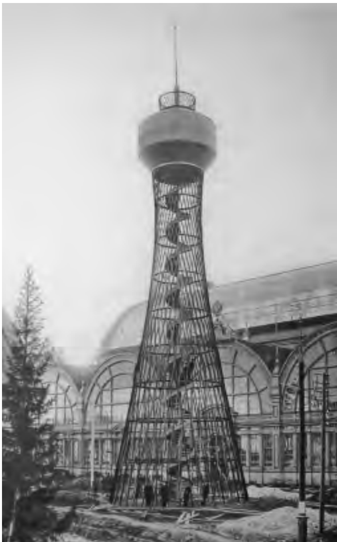
The world's first hyperboloidal design Water tower. Nizhny Novgorod, 1896
