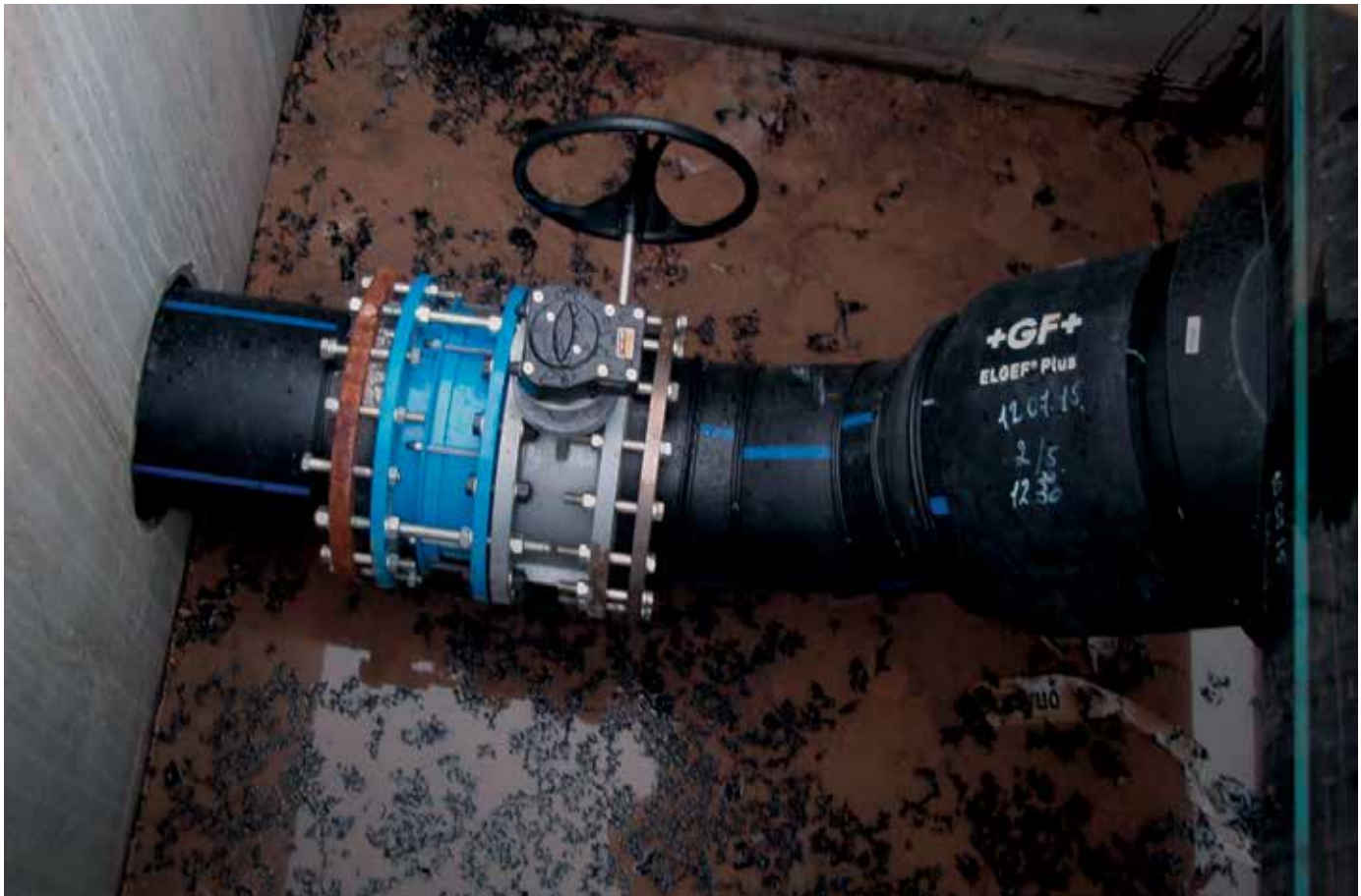
Pic. 3. Completed branch
