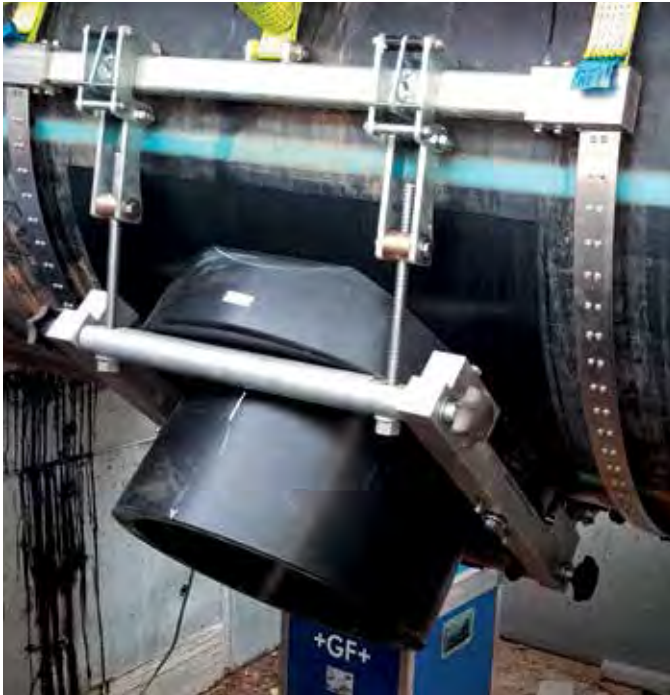
Pic. 2. Saddle positioning onto the pipes
