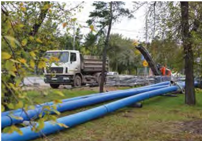
The construction work was carried out using the open trench method. Several areas required horizontal directional drilling and PROTECT pipes with a PP protective coating were used.
