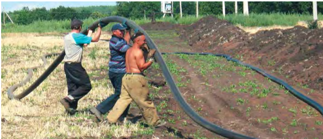
Pic. 3. Oil flowline positioning
