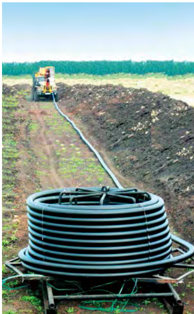
Pic. 2. Uncoiling of Anaconda™ pipe during construction of oil flowline
