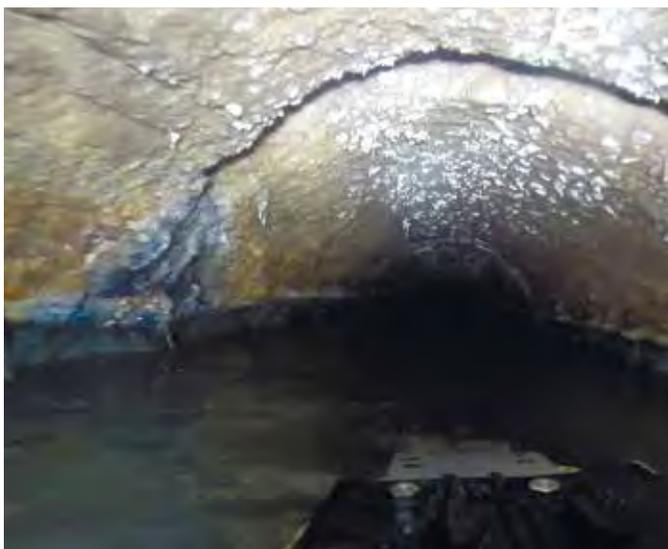
**Pic. 2. Opening of the crown of pipelines**
