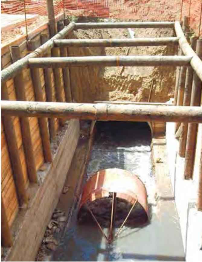
**Pic. 3. Pipelines bottom cleaning**
