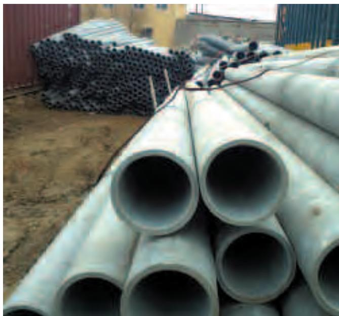
Asbestos pipes are gradually being replaced by plastic or other safer pipes in Podgorica. Over 150 km of water pipelines were installed within the last few years using modern materials and new technologies.
