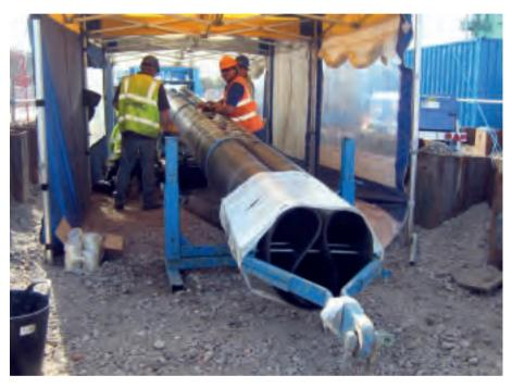
The pipe can be reduced on site during installation or can be prepared inhouse beforehand. The liner is installed using the sliplining process, and the reduced diameter pipe is pressurised allowing it to revert to its original size, forming a close fit within the host pipe. The range of pipe diameters is from 100 mm to 500 mm, with nominal pressure up to PN16. Installation of up to 1.5 km in a single insertion is possible.
