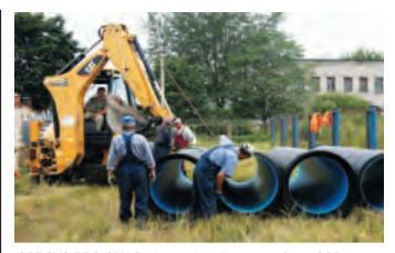
CORSYS PRO SN16 pipes with diameters from 200 mm to 630 mm were supplied to the project. Currently negotiations are being held regarding further pipe supplies to Petrolesport OJSC.
