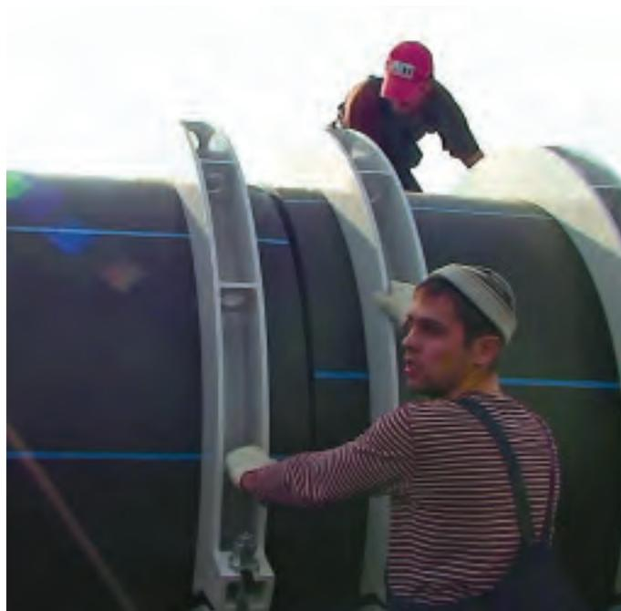
nected and lowered onto the seabed (to a depth of 34 metres). The unique pipeline lowering operation was successful and the pipes and connections demonstrated excellent strength and flexibility by withstanding significant bending loads during the installation.
