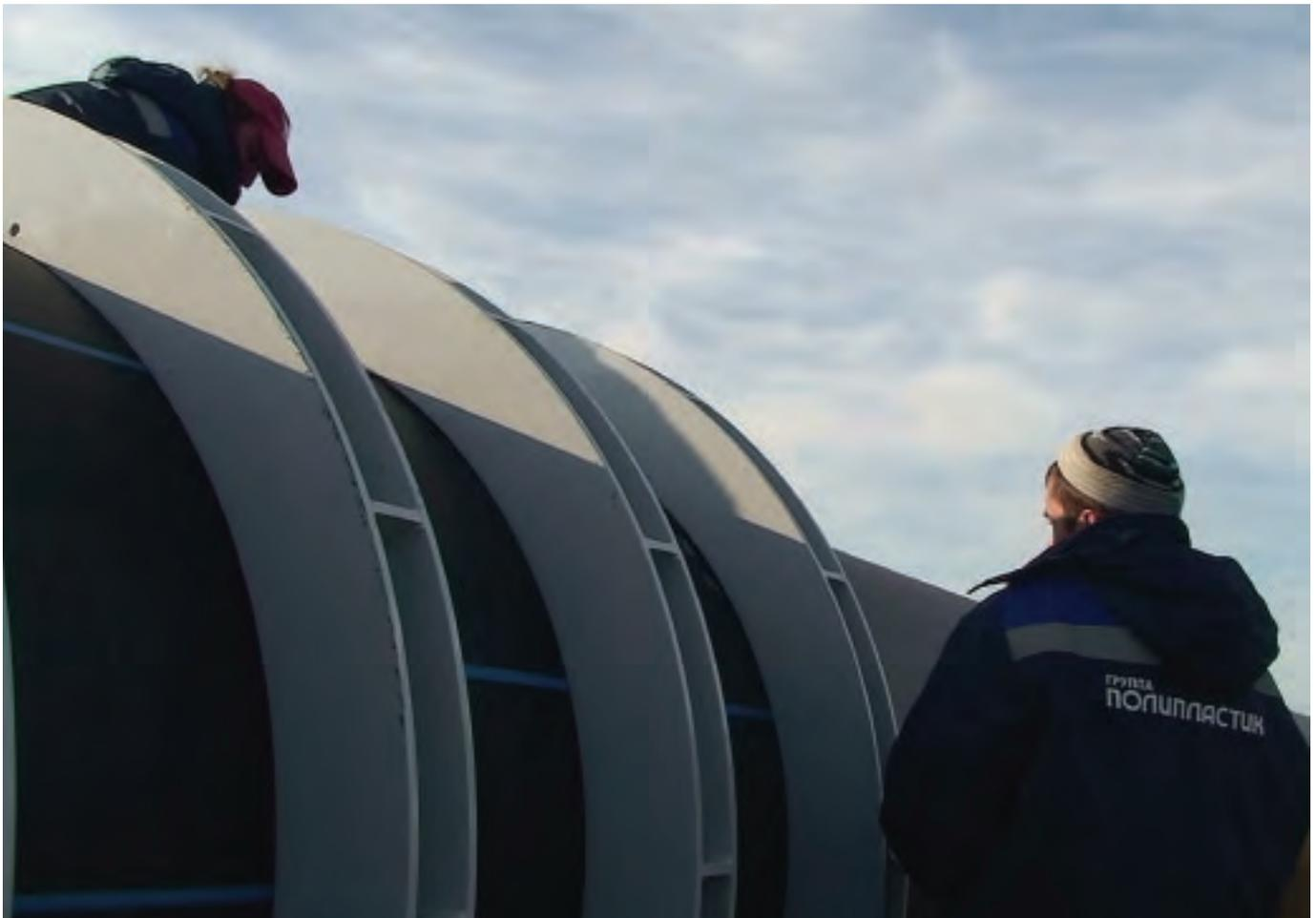
and tilting, and branch pipes had to be stiffened to withstand jet thrust load.
