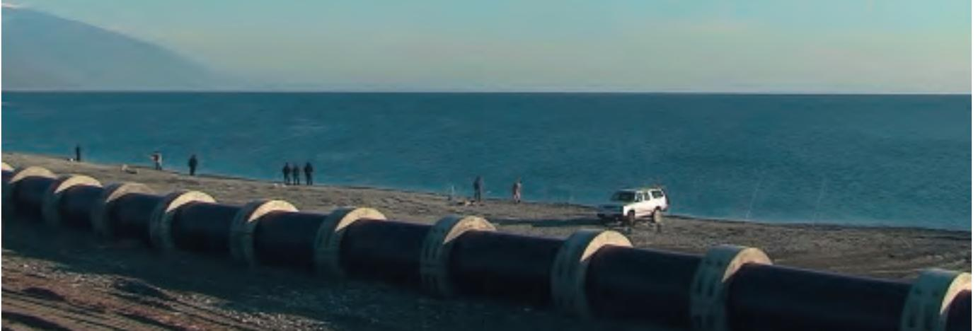
In the summer of 2011, POLYPLASTIC Group began producing PE pipes up to 1600 mm in diameter at the Klimovsk Pipe plant. The first large-scale project involving these 1600 mm pipes was the Olympic facility in Sochi.
