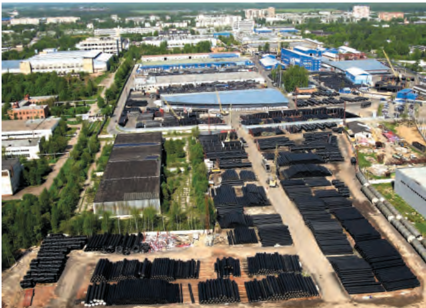
Klimovsk pipe plant site: summer 2008
